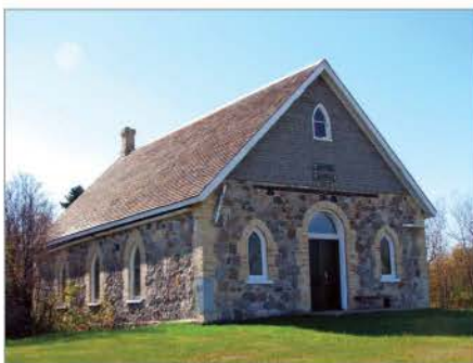
FIG. 13. VIEW OF THE WEST FAÇADE OF POPLAR GROVE PRESBYTERIAN CHURCH, UNKNOWN ARCHITECT. | KRISTIE DUBÉ.
