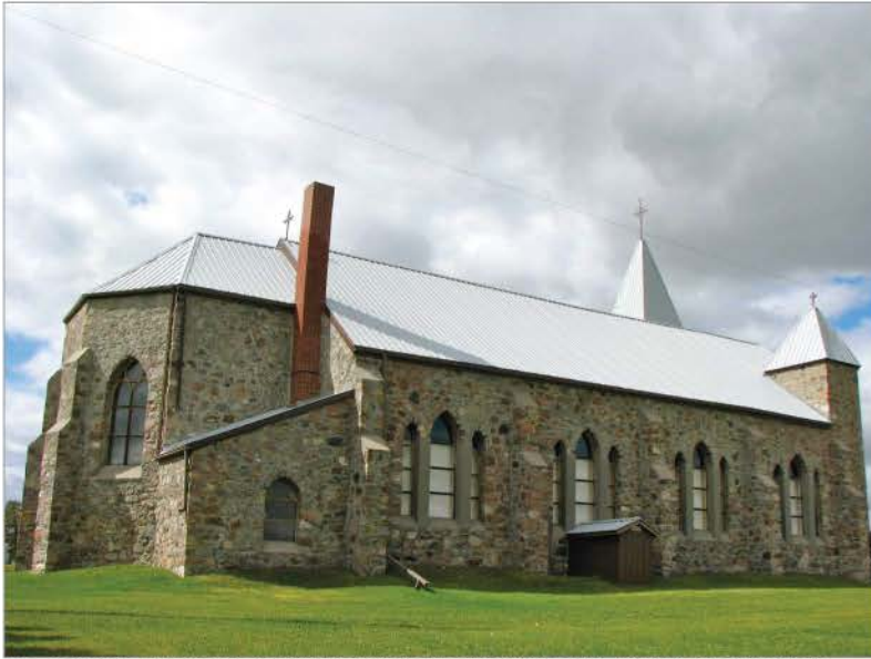
FIG. 4. VIEW OF EASTERN AND NORTHERN SECTIONS SHOWING HEXAGONAL CHANCEL AND ABA LANCET TRIPARTITE WINDOWS, KAPOSVAR ROMAN CATHOLIC CHURCH, KAPOSVAR, RM 183. | KRISTIE DUBÉ.
