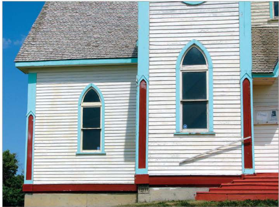
FIG. 15. DETAIL OF GABLETS MIMICKING MASONRY BUTTRESSES, BEKEVAR PRESBYTERIAN CHURCH, BEKEVAR, RM 94. | KRISTIE DUBÉ.
