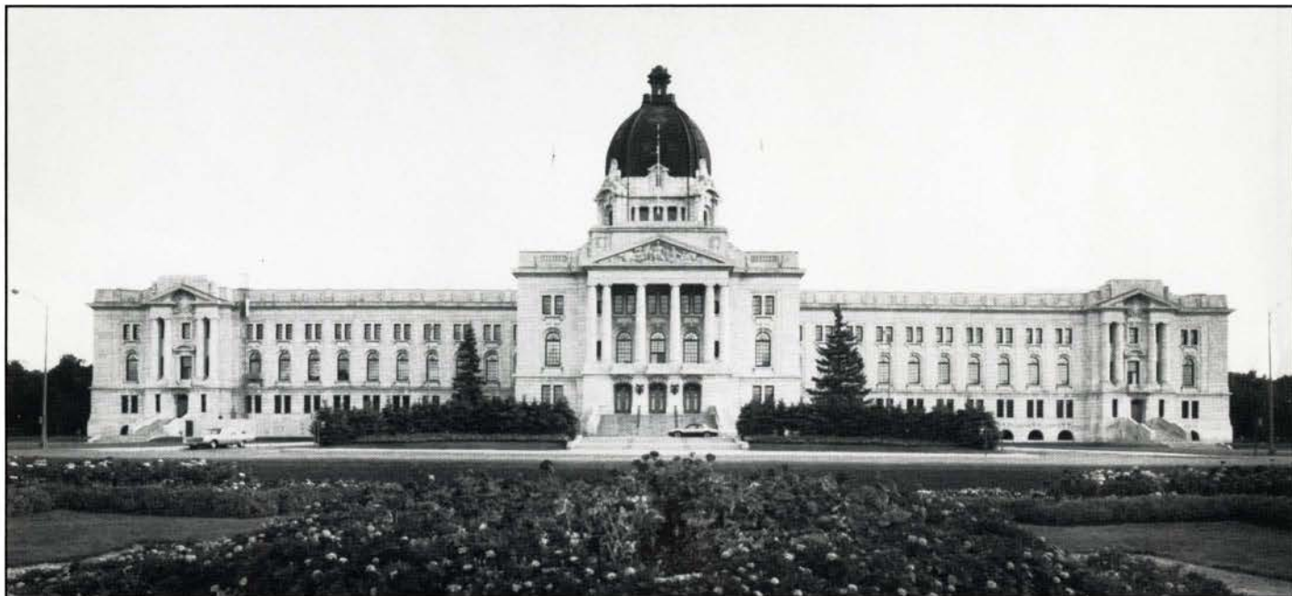
Saskatchewan Legislative Building, E. and W.S. Maxwell, architects, 1907-12.
