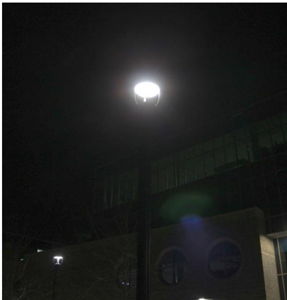
Figure 5 Example of uni-directional lighting in the Steele Ocean Sciences Building parking lot. Note the inset light bulb and the effectiveness of the top cover.
