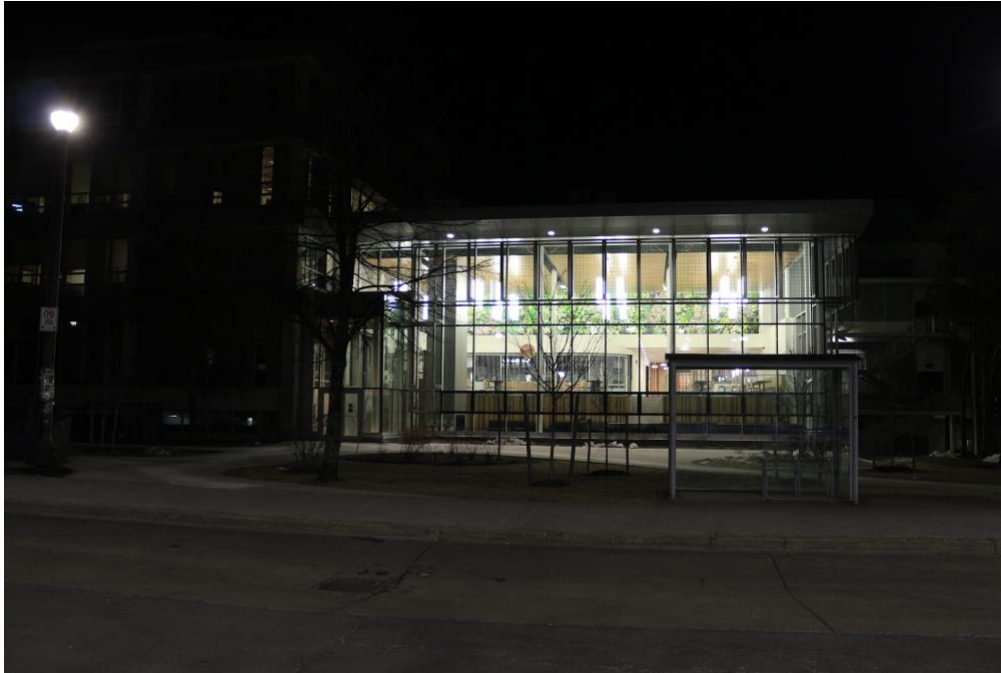
Figure F3 The Student Union Building extension at night on March 27, 2018 at Dalhousie University's Studley campus.
