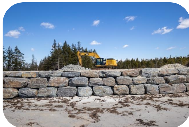
Privitization along the coastline, building of a sea wall. Photo by: Nicolas Winkler
