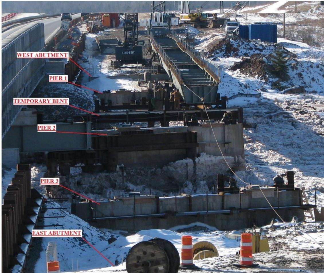
**Figure 3.1: Halifax bound structure during construction (north girder shown)**
